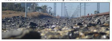
Due to the selective bonding of stones at contact points the drainage capacity of the ballast will be fully maintained even during heavy rainfall.
